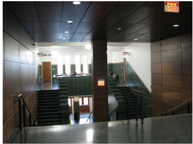
Figure 7. Looking east to west from the new addition to the third level of the original structure.
