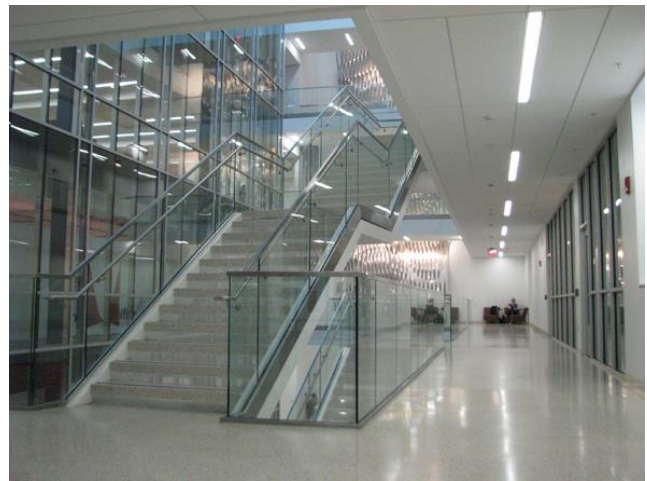
Figure 8. Juxtaposition of volumes between the central atrium void and circulation paths in the new addition.
